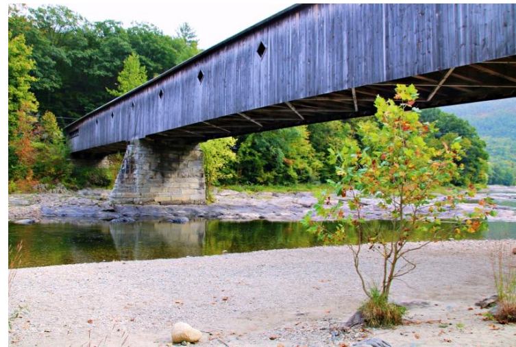
Williamsville Covered Bridge
